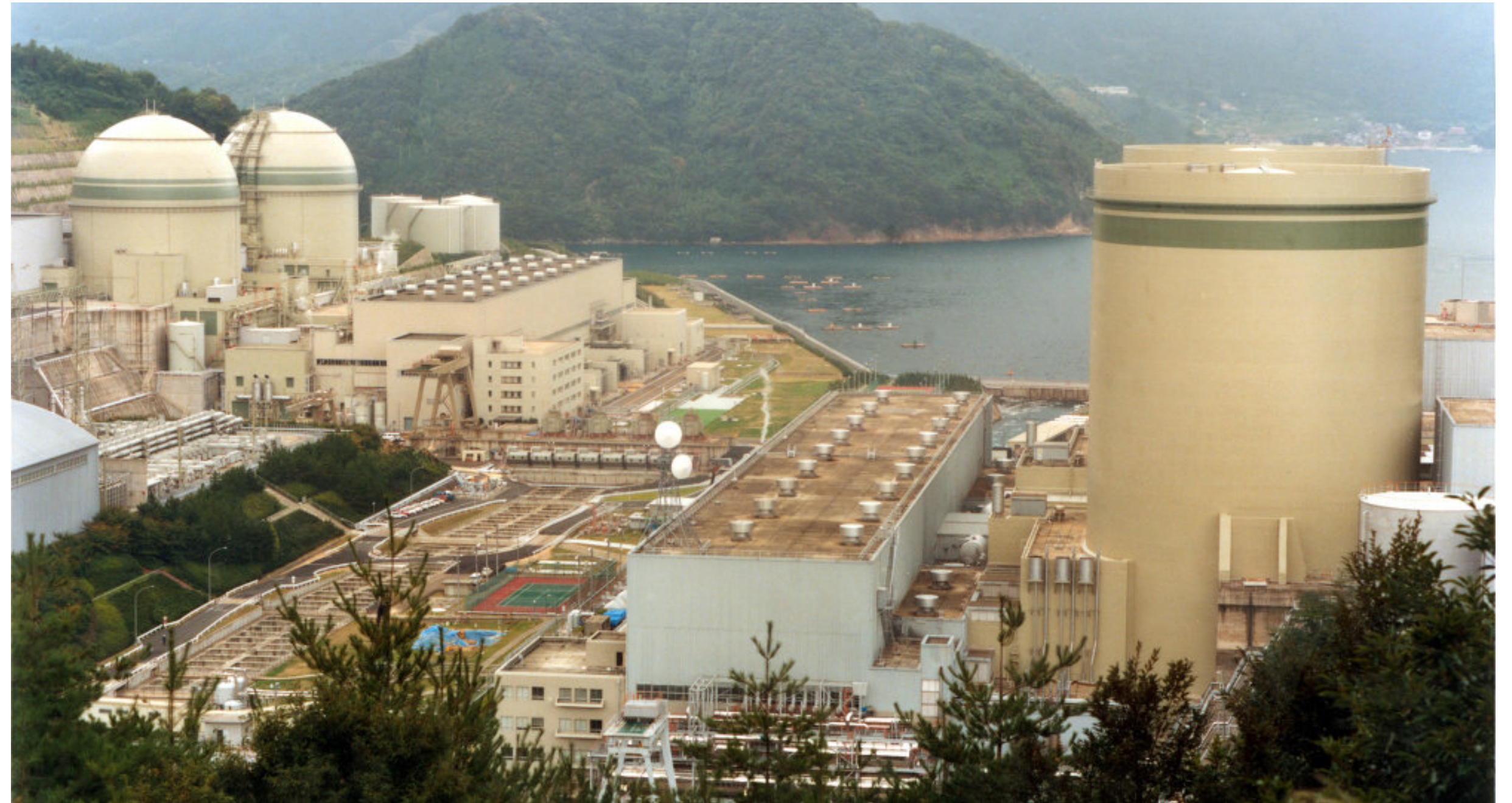
Takahama Nuclear Plant
