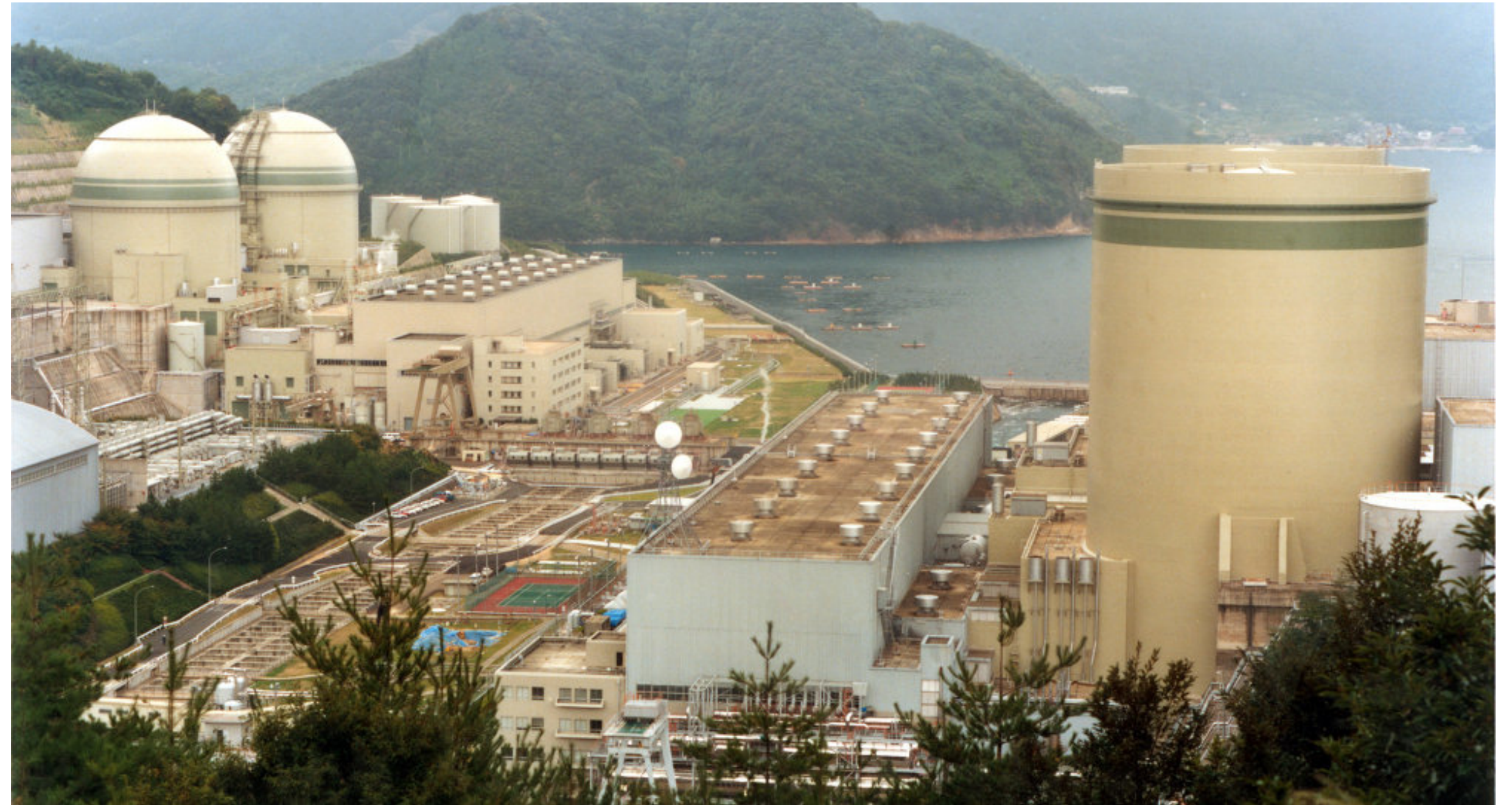
Takahama Nuclear Plant
